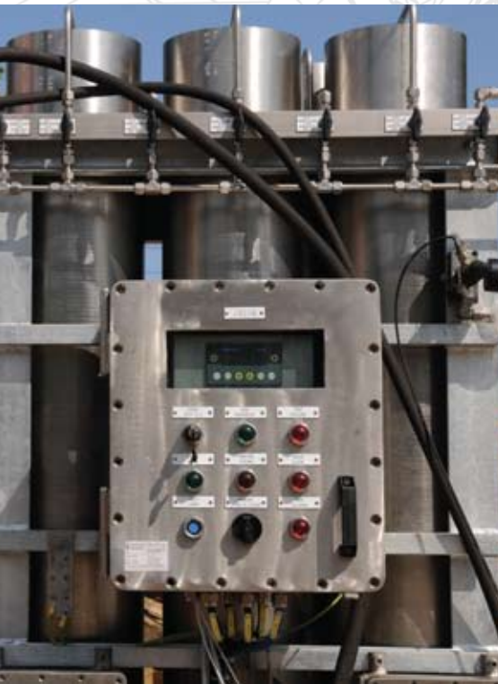
SSIV Control System - Topside Umbilical Terminal Unit (TUTU) c/w Hydraulic Power Unit TUNA Gas Gathering PLEM and SSIV System Project (Egypt) - PETROBEL
