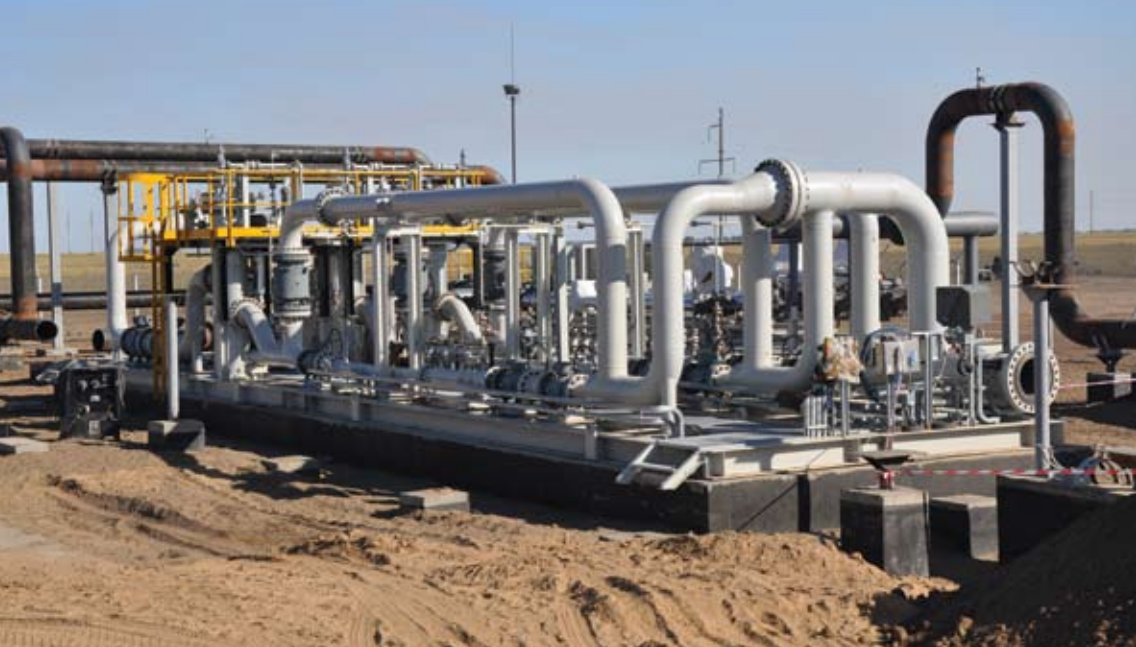
Gas Pressure Reducing Station Karachaganak - Uralsk Gas Pipeline Project (Kazakhstan) KPO
