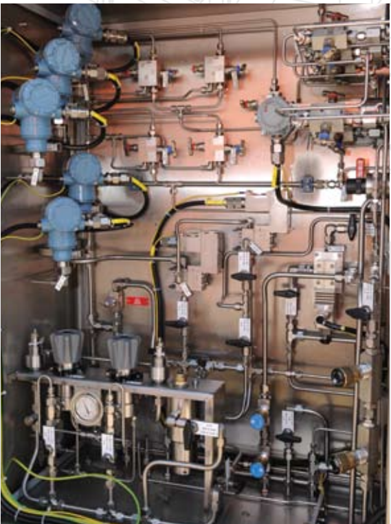
SSIV Control System - Topside Umbilical Terminal Unit (TUTU) c/w Hydraulic Power Unit TUNA Gas Gathering PLEM and SSIV System Project (Egypt) - PETROBEL
