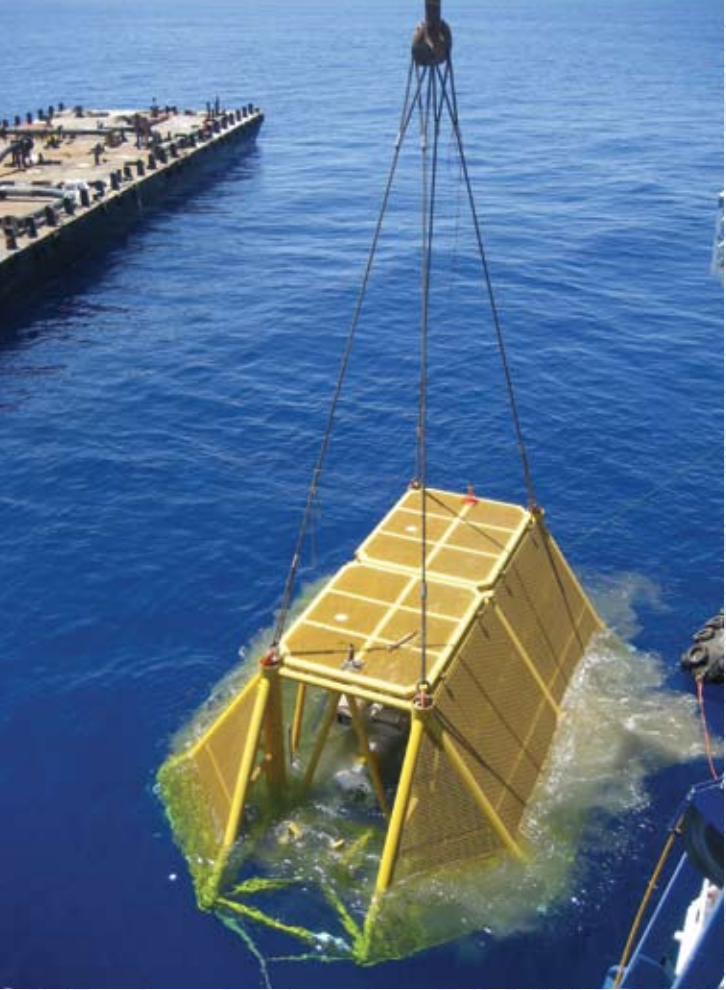
Deployment of PLEM to sea-bed TUNA Development Project (Egypt) - PETROBEL
