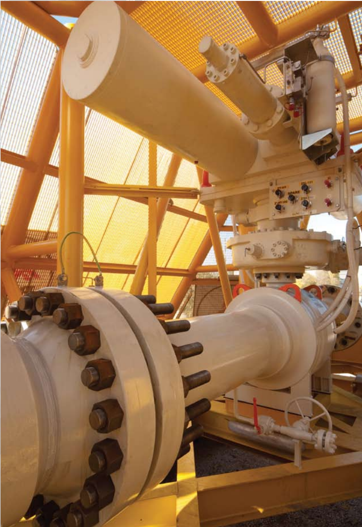
SSIV Station - 24" Hydraulically Actuated Ball Valve TUNA Gas Gathering PLEM and SSIV System Project (Egypt) - PETROBEL
